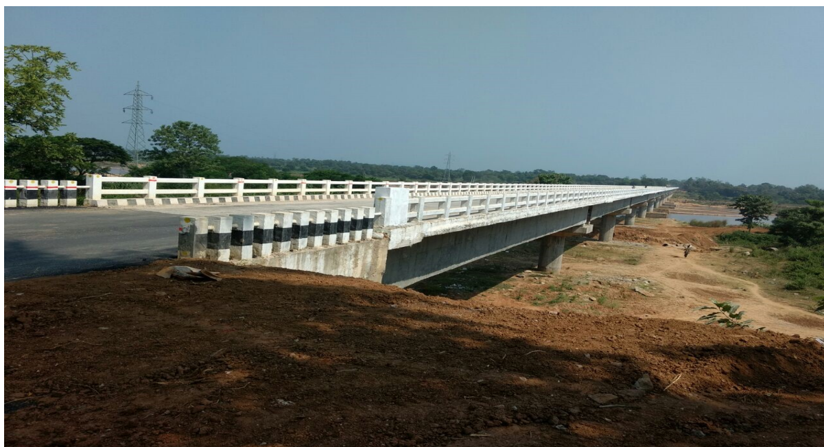
Sample Photo: High level bridge constructed over river Vansadhara of Gumuda – RIDF Project
